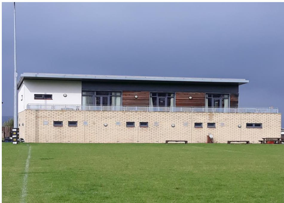
Figure 1 – Image of the exterior of Greenock Wanderers' clubhouse
